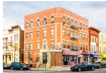
Under Contract – Fox Street 9,920 SF - 13 Units
