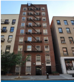
402 East 83rd Street
